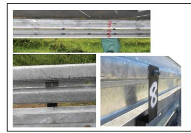
MPS Fixture bracket (24.70) to be fixed to the barrier at hole 1.00 m and 3.00 m (barrier with 1 m punching necessary).
