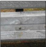
beam with 1 HRK M16x40, 4.6 with nut (40.01) and washer 18 (40.30) and butt plate M16 (10.00)
